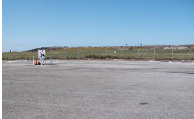
Figure 5: Post-construction Station Image
